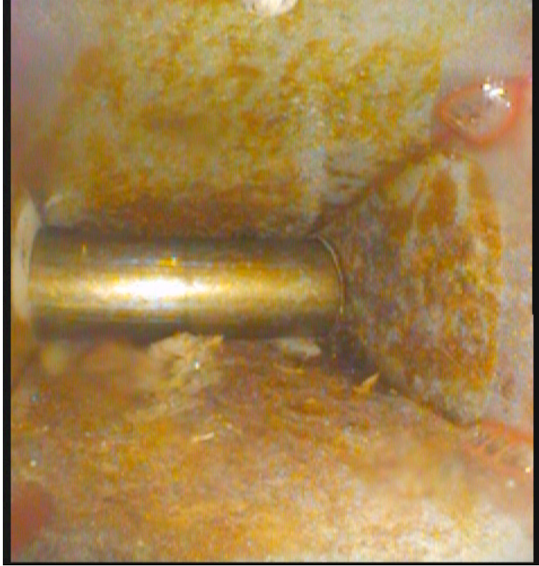
Fig. 4 Borescope View - Inside Center Lug Cavity
